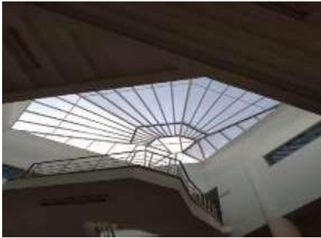
Building of the Institutes
